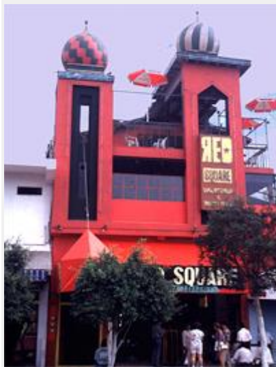
Playful architecture along Revolution Avenue in downtown Tijuana emerged during the NAFTA era of economic growth in the 1990s (photo by L. Herzog)
